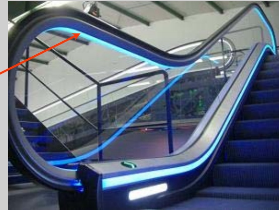
LED Balustrade lighting
