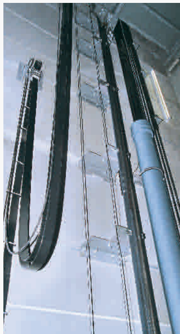
Shaft height section of a hydraulic drive freight elevator
